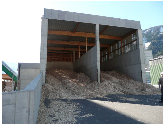
Figure IV.A.3-2: Automatic fuel storage facility with two push floor units
