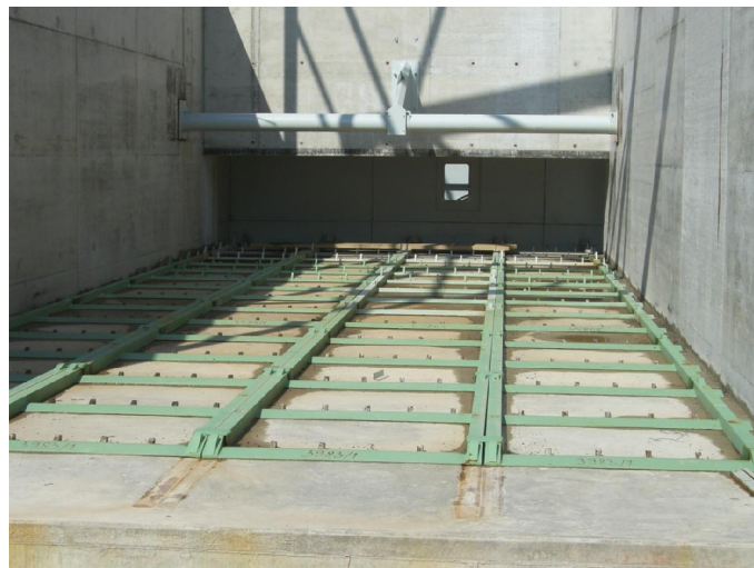
Figure IV.A.3-1: Push floor unit before operation
